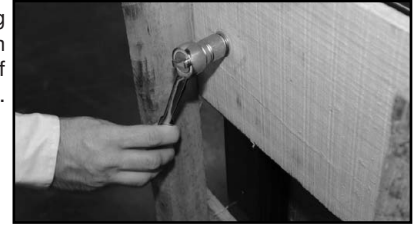
Removing skid from bottom of cabinet.
