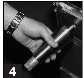
4 Thread leg into cabinet bottom frame rail.
