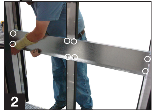
2 Bracket removal. Thumb screw locations.
