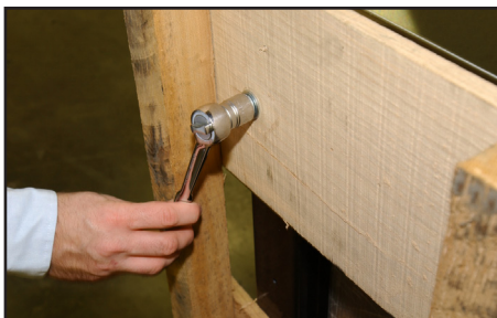
Removing skid from bottom of cabinet.
