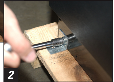
2 Removing bracket from cabinet.
