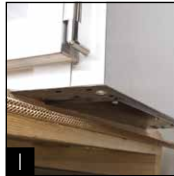
Slide packing material under the unit.
