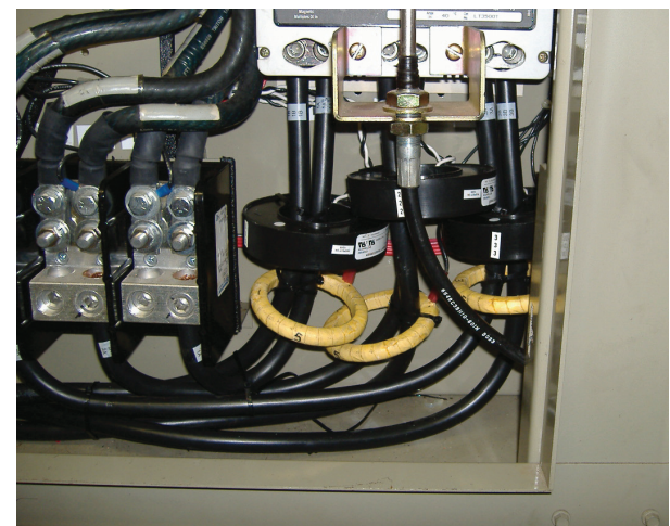
Figure 39. RTHD - Installation of CTs
