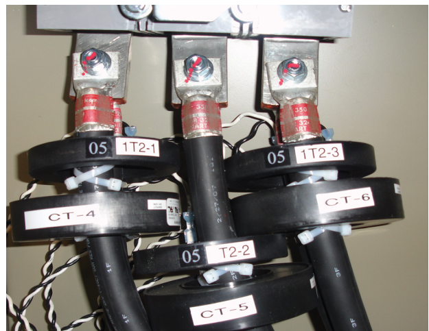
Figure 39. RTHD - Installation of CTs
