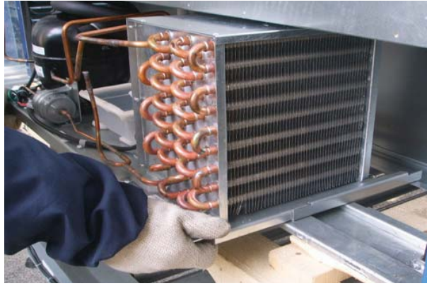
B. Disassembly the condensing unit
