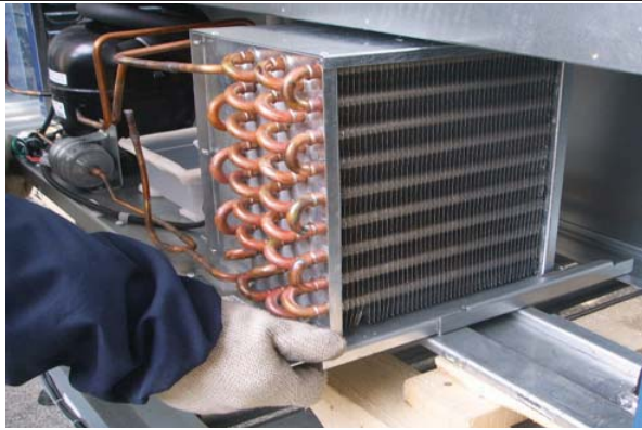
B. Disassembly the condensing unit
