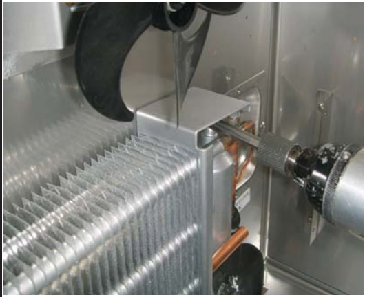
A.Remove the evaporator coil
