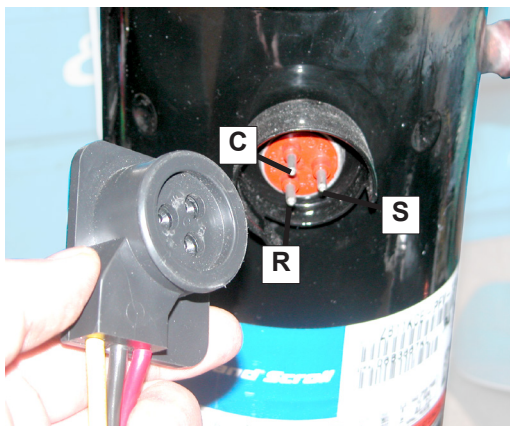
Figure 3-3 Compressor Connection
