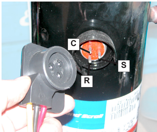
Figure 3-3 Compressor Connection
