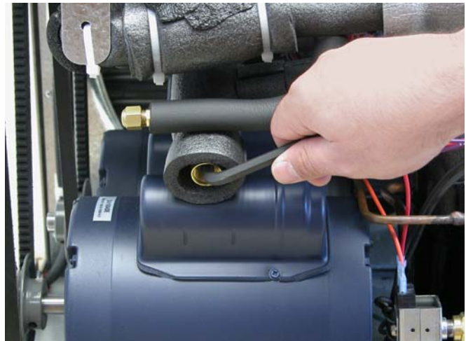
Figure 5-8 Hot Gas Bypass Adjustment
