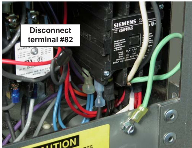
Figure 5-2 Disconnect Compressor Coil
