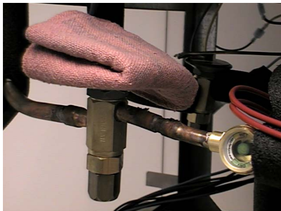
Figure 5-5 TXV Removal
