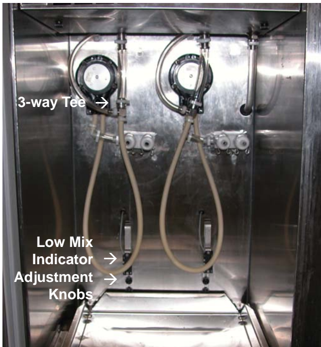
Figure 2-6 Connecting Pump Hose to BCS Manifold
