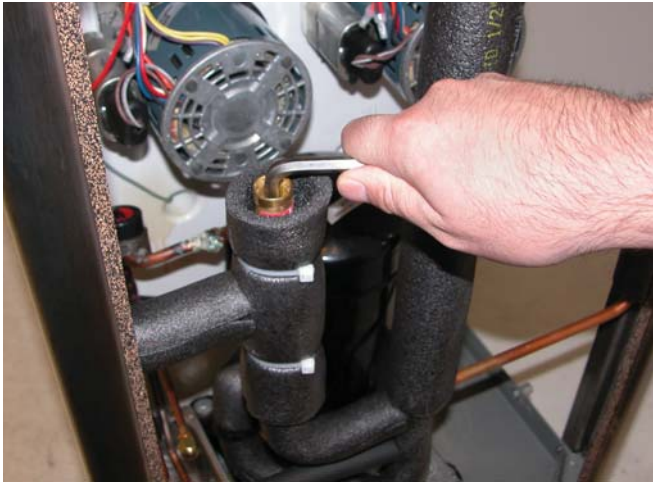
Figure 5-8 Hot Gas Bypass Adjustment
