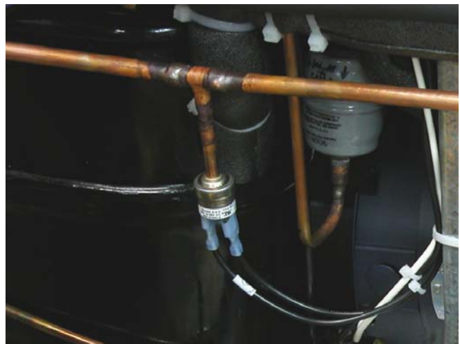
Figure 5-6 High Pressure Cutout
