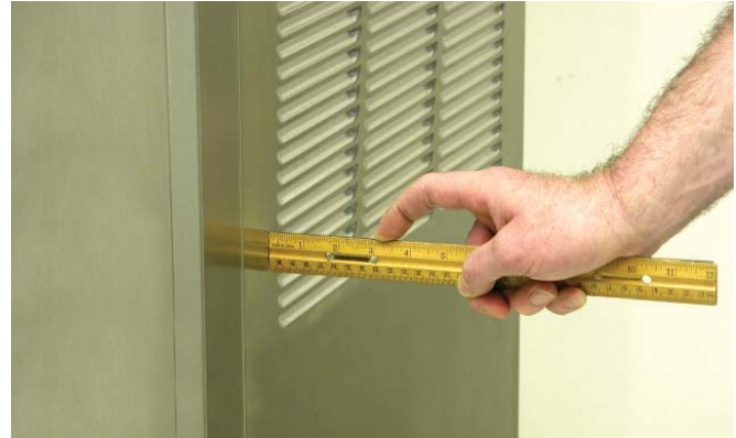
Figure 2-1 Space and Ventilation Requirements
