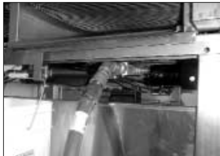
N724/750 Equipment Side Gas Connection
