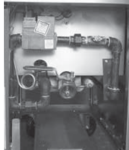
Gas valve in the RF40.
