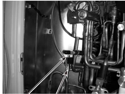
Bypass valve fixing screw
