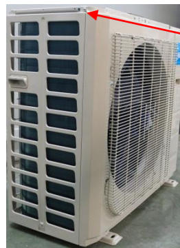
Screws of front panel
