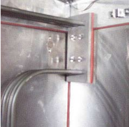
FIG. 45 Heating Element with Gasket & Fasteners
