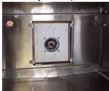
FIG. 35 Motor with Motor Mount Bracket
