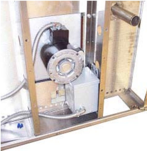
FIG. 39 Transformer
