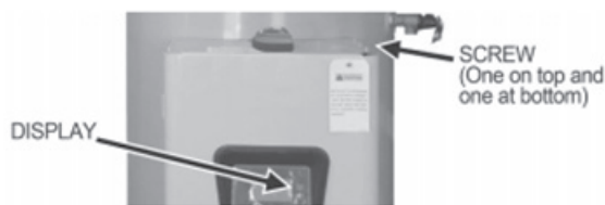
Figure 14. Loosening the Screws to the Door of the Unit
