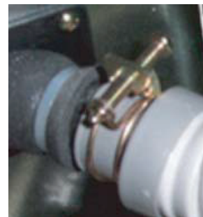
Figure 87: Flexible Drain Hose Connection.
