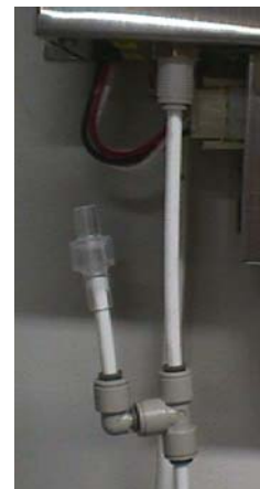
Siphon Break Installation Figure 2
