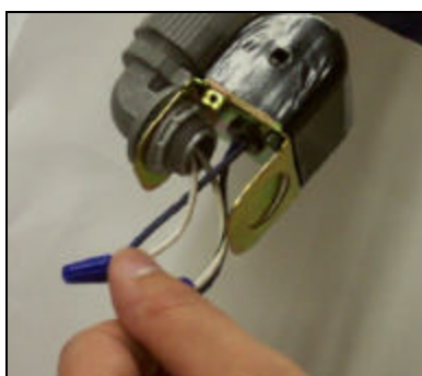
Straightening the wires
