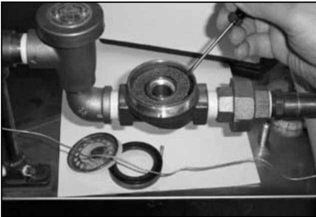
Removing the mesh strainer screen
