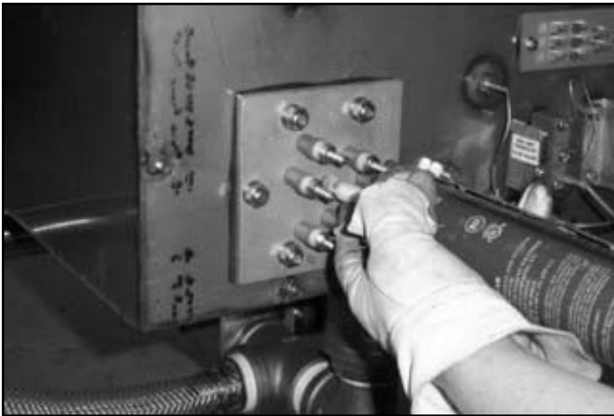
Applying silicone to the heater well
