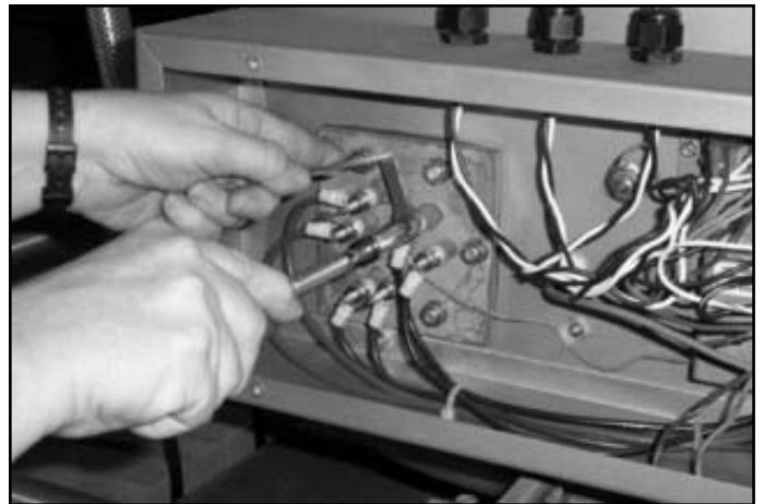
phase operation tightening the nuts holding the power lines
