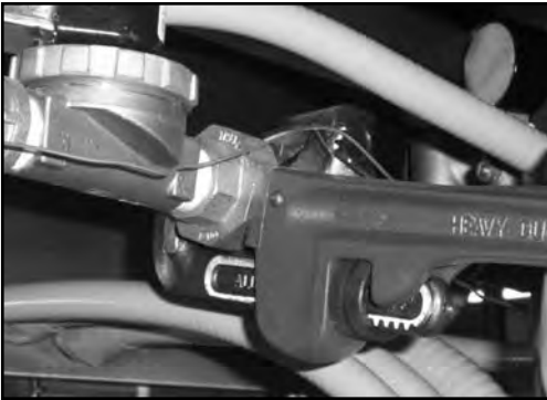
Loosening the union on the incoming plumbing
