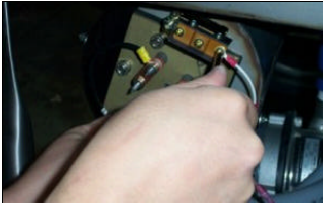
Securing jumpers to the thermostat.
