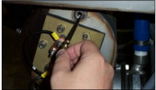
Pulling the thermostat probe and fitting from the well (Tempstar).
