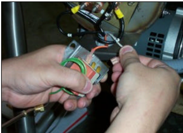
Removing the wires from the thermostat.
