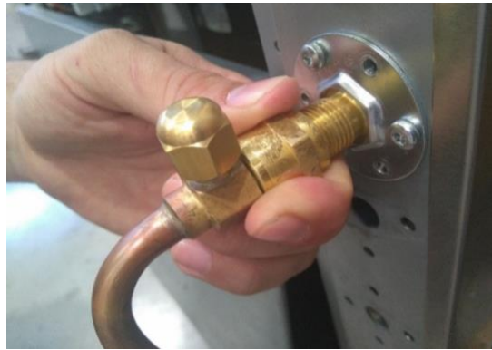
Picture 6: Thread the couplings by hand
