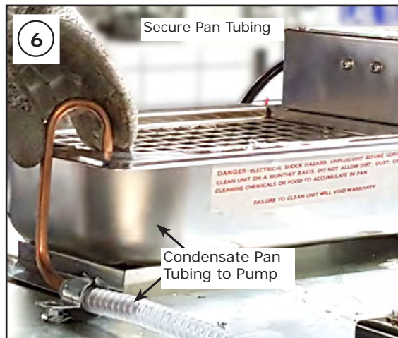
Condensate Pan (Installed on top of case)
