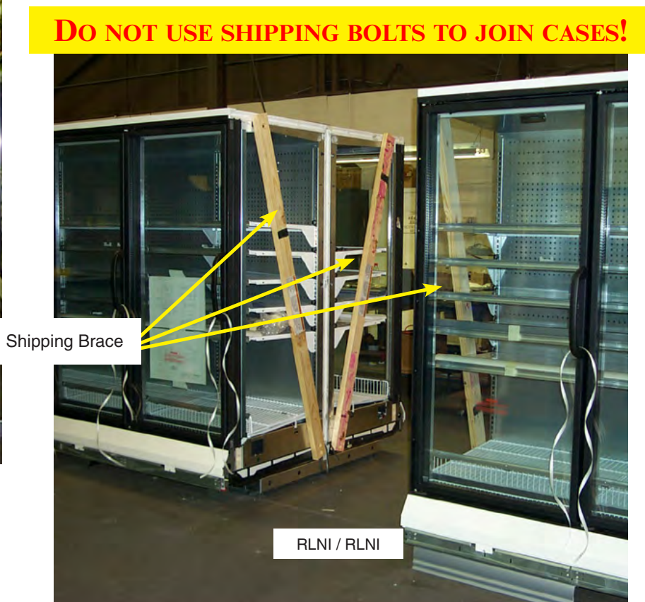
Figure 3. Remove Shipping Braces
