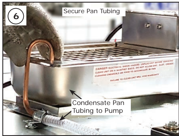
Condensate Pan (Installed on top of case)
