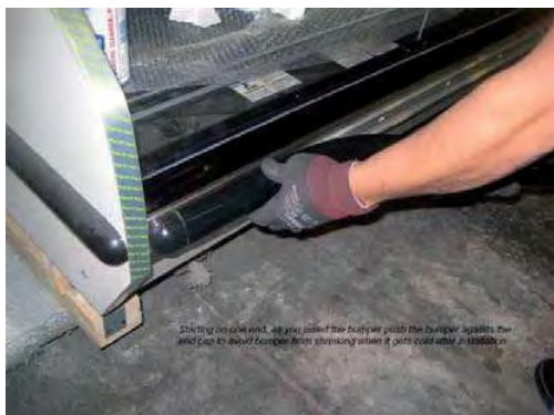
Step 3: Starting on one end: while inserting the bumper, push it up against the end cap to prevent the bumper from shrinking after installation (when it gets cold).
