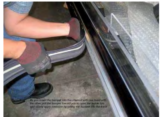
Step 4: As you insert the bumper into the channel with one hand, pull the bumper toward you with the other to open the inside lips. Slowly apply pressure by rolling the bumper into the track.
