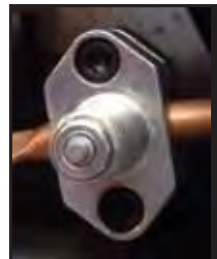
refrigeration line tapping valve
