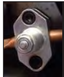
refrigeration line tapping valve
