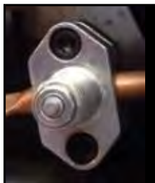
refrigeration line tapping valve
