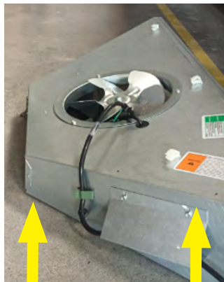
Lift up Fan Plenum. Use chain to hook up fan plenum to facilitate cleaning.
