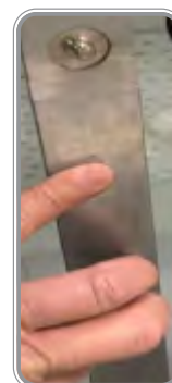
Attach template to door over existing stud location. Use tape or clamp to secure.
