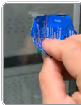
Wipe the area where the stud goes with a towelette. Allow to dry for 1 minute. Do not touch glass again.
