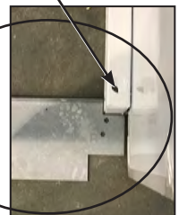
Drill hole through base upright into floor.
