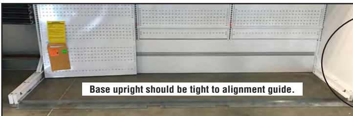
Drill hole through base upright into floor.
