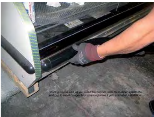
Step 3: Starting on one end: while inserting the bumper, push it up against the end cap to prevent the bumper from shrinking after installation (when it gets cold).
