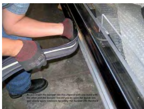
Step 4: As you insert the bumper into the channel with one hand, pull the bumper toward you with the other to open the inside lips. Slowly apply pressure by rolling the bumper into the track.
