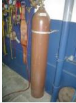
DRY NITROGEN TANK
