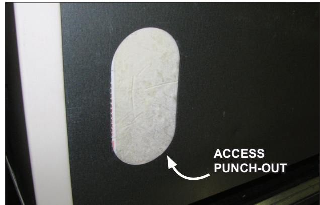
Fig. 11 Penetrate foam as needed to access piping
