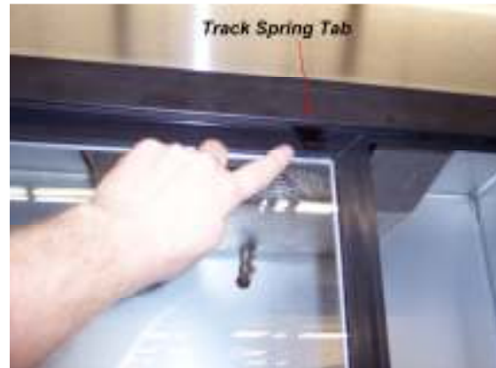
Figure 8. Door Track Spring Tab.
