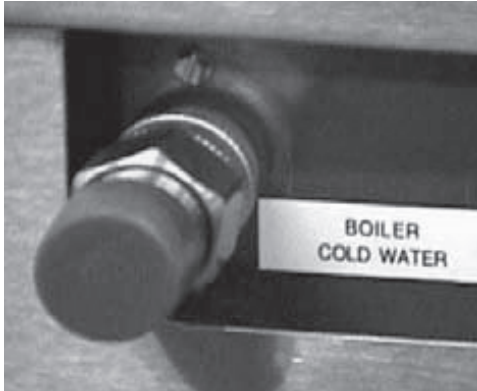
The BPST Connection on the right rear side of the steamer.
