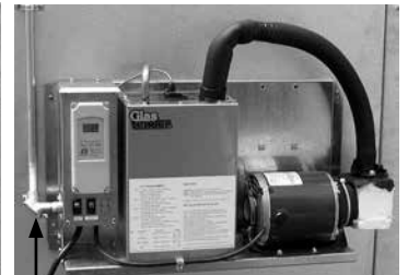
Install power line between condensing unit and control panel.
