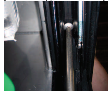
[Photo 5– Upper Track View]
