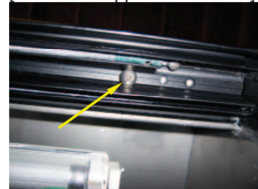
[Photo 4 – Upper Track View]
