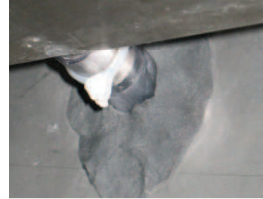
Install new drain pan. Insert drain tube thru hole - downward angle
