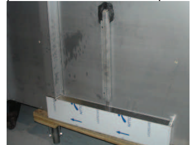
Install rear drain tubing chase to hold elbow at bottom of hole & ensure a drain downward slope.
