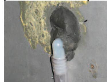
Install elbow, push to bottom of hole and secure with sealant.
